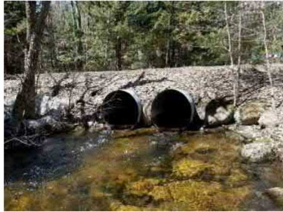
Dry-laid stone outlet headwall
