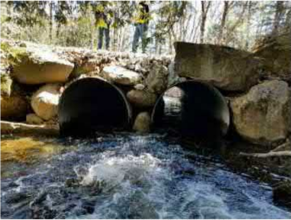
Dry-laid stone inlet headwall
