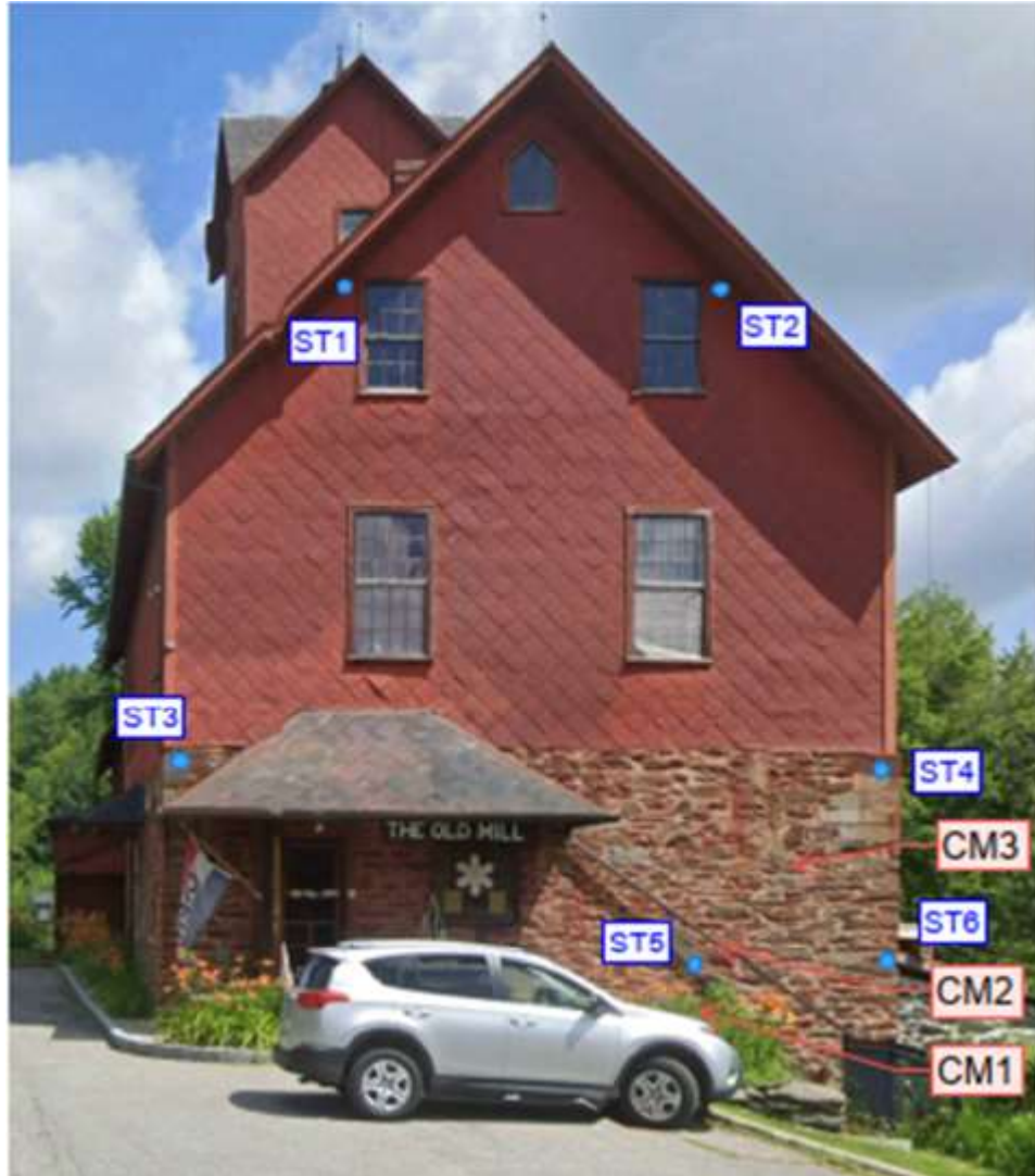
Image 1: Approximate location of survey targets (ST-#) and crack monitors (CM-#)
