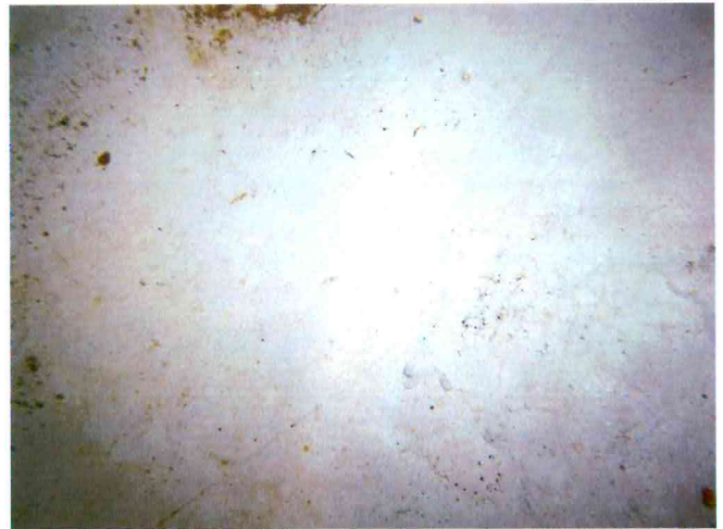
38 Floor Surfaces Found With Coating Failure, Exposed Steel, Moderate Surface Corrosion And Pitting After Cleaning
