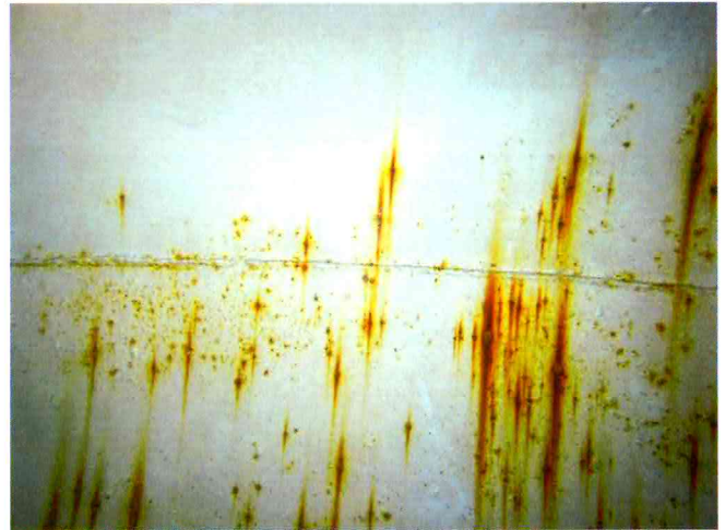
52 Interior Wall Panels Found With Coating Failure, Exposed Steel, Moderate Surface Corrosion And Pitting
