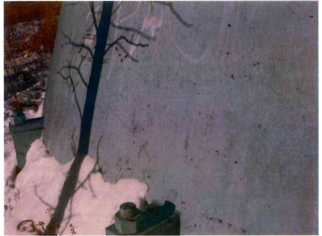
2 Exterior Wall & Bowl Surfaces Found With Nearly Expired Chalky Coating, Chips Throughout Lowest 30' Of The Pedestal And Mildew Throughout The Underside Of The Bowl
