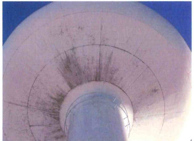
10 Exterior Wall & Bowl Surfaces Found With Nearly Expired Chalky Coating, Chips Throughout Lowest 30' Of The Pedestal And Mildew Throughout The Underside Of The Bowl
