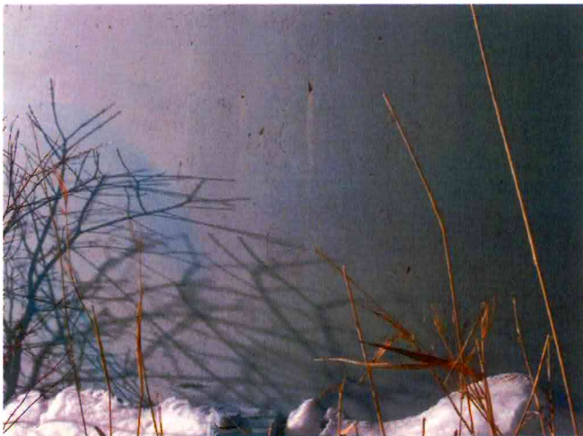
3 Exterior Wall & Bowl Surfaces Found With Nearly Expired Chalky Coating, Chips Throughout Lowest 30' Of The Pedestal And Mildew Throughout The Underside Of The Bowl
