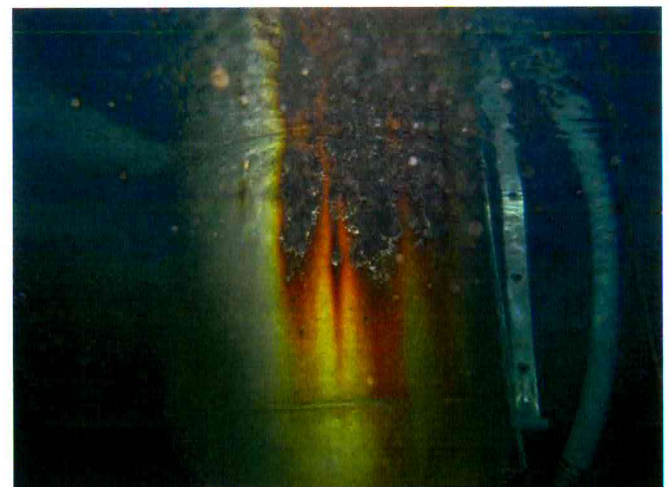
66 Center Riser Column Found With Coating Failure, Exposed Steel And Moderate Surface Corrosion
