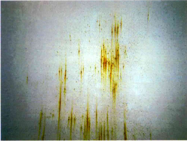
61 Interior Wall Panels Found With Coating Failure, Exposed Steel, Moderate Surface Corrosion And Pitting
