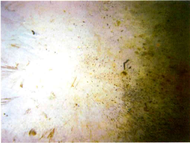
37 Floor Surfaces Found With Coating Failure, Exposed Steel, Moderate Surface Corrosion And Pitting After Cleaning
