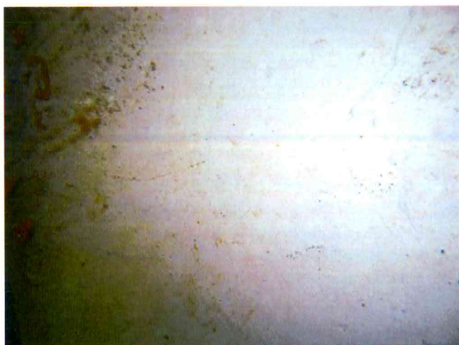
41 Floor Surfaces Found With Coating Failure, Exposed Steel, Moderate Surface Corrosion And Pitting After Cleaning
