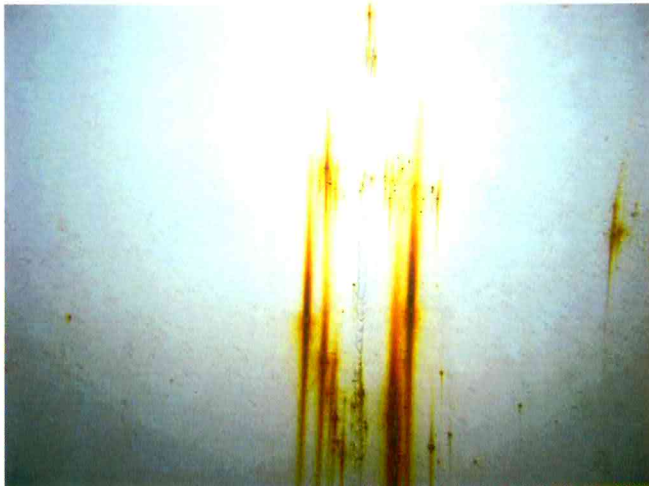
51 Interior Wall Panels Found With Coating Failure, Exposed Steel, Moderate Surface Corrosion And Pitting
