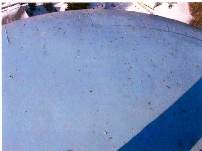
27 Roof Panels Found With Nearly Expired Chalky Coating
