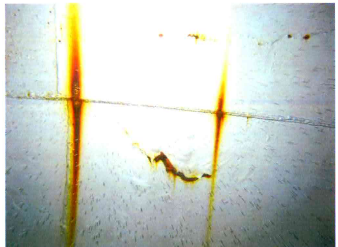
54 Interior Wall Panels Found With Coating Failure, Exposed Steel, Moderate Surface Corrosion And Pitting
