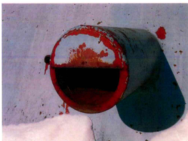
23 Unscreened Overflow Pipe
