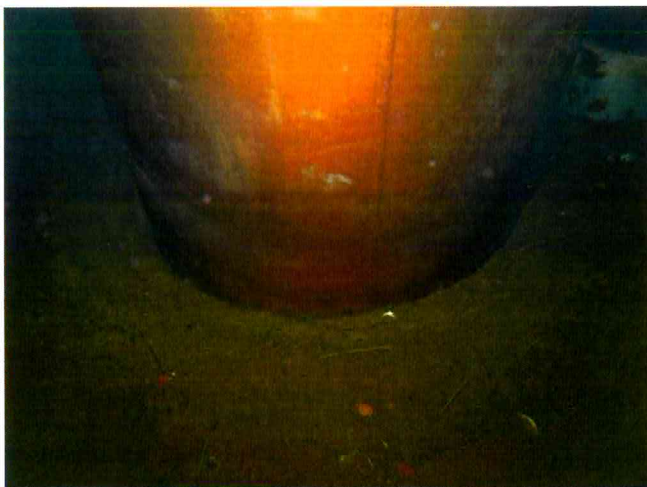
65 Center Riser Column Found With Coating Failure, Exposed Steel And Moderate Surface Corrosion
