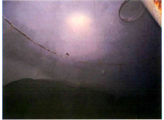
68 Overhead Panels Found With Coating Failure And Blotch Rusting
