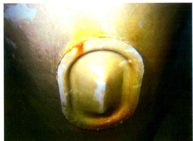
42 Manway Found With Coating Failure, Exposed Steel And Moderate Surface Corrosion
