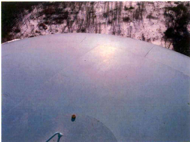
25 Roof Panels Found With Nearly Expired Chalky Coating
