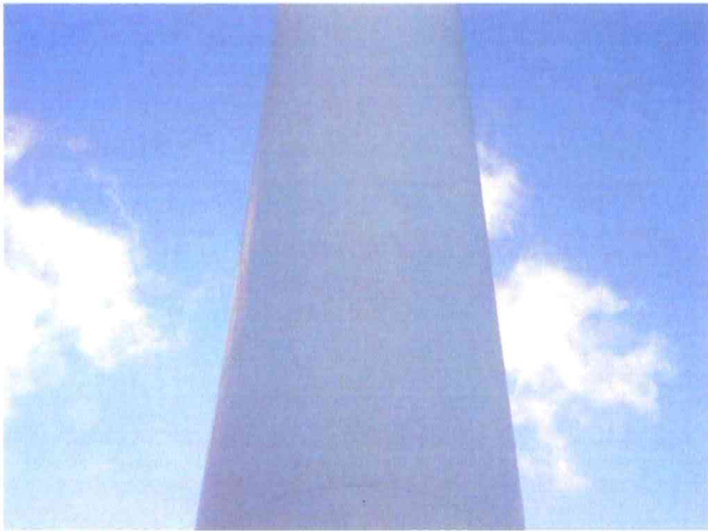
7 Exterior Wall & Bowl Surfaces Found With Nearly Expired Chalky Coating, Chips Throughout Lowest 30' Of The Pedestal And Mildew Throughout The Underside Of The Bowl
