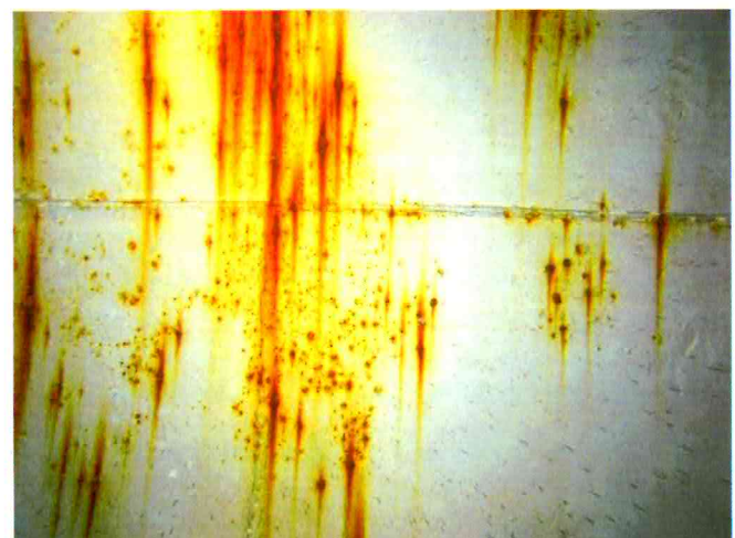
48 Interior Wall Panels Found With Coating Failure, Exposed Steel, Moderate Surface Corrosion And Pitting
