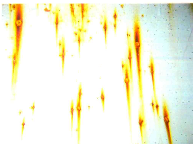
59 Interior Wall Panels Found With Coating Failure, Exposed Steel, Moderate Surface Corrosion And Pitting
