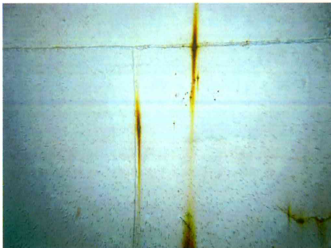
53 Interior Wall Panels Found With Coating Failure, Exposed Steel, Moderate Surface Corrosion And Pitting
