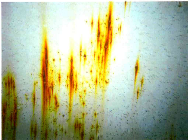
45 Interior Wall Panels Found With Coating Failure, Exposed Steel, Moderate Surface Corrosion And Pitting
