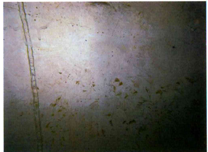
40 Floor Surfaces Found With Coating Failure, Exposed Steel, Moderate Surface Corrosion And Pitting After Cleaning
