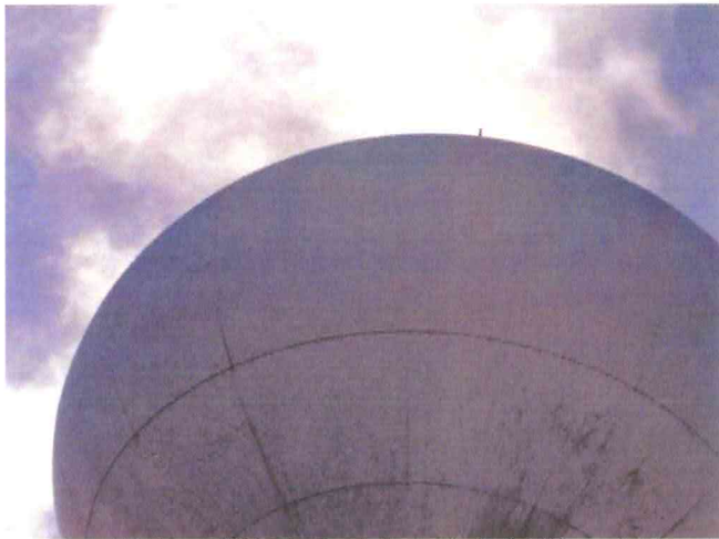
13 Exterior Wall & Bowl Surfaces Found With Nearly Expired Chalky Coating, Chips Throughout Lowest 30' Of The Pedestal And Mildew Throughout The Underside Of The Bowl
